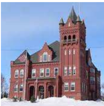
The Wayne County Court House in winter, Wayne, Nebraska
