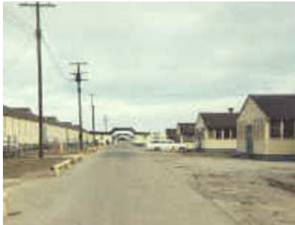
Fort Leonard Wood road and barracks in the 1960's.
