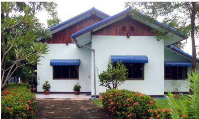
The Sam and Gan Burris house in Na Ku, Kalasin Province, Thailand. Sam's "Virginia porch swing" is on the left side. The kids room, which was Mama's previously, is located on the right with a large common room is in the center, 2009.
